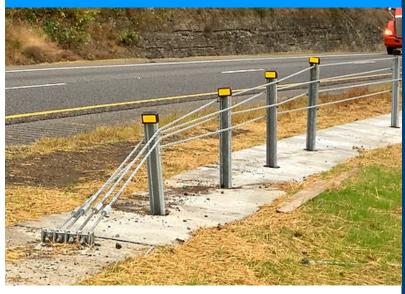
For more Information ContactThis Z shaped post design has the top rope in a U-channel and the 3 woven lower ropes positioned on the posts with the use of nylon pegs allowing the high rope to post friction created during crashes to control the deflection of impacting vehicles. The woven rope design improves system performance and ease of maintenance while providing predictable deflections regardless of length between terminals.
